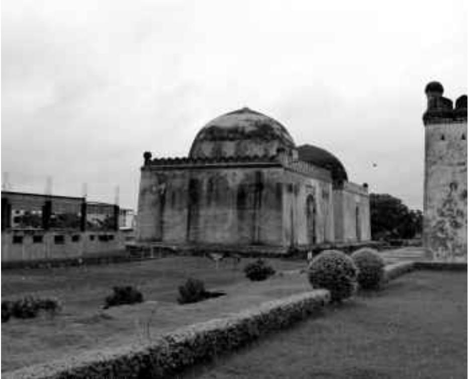
Figure 5. Haft Gumbaz complex, Gulbarga
