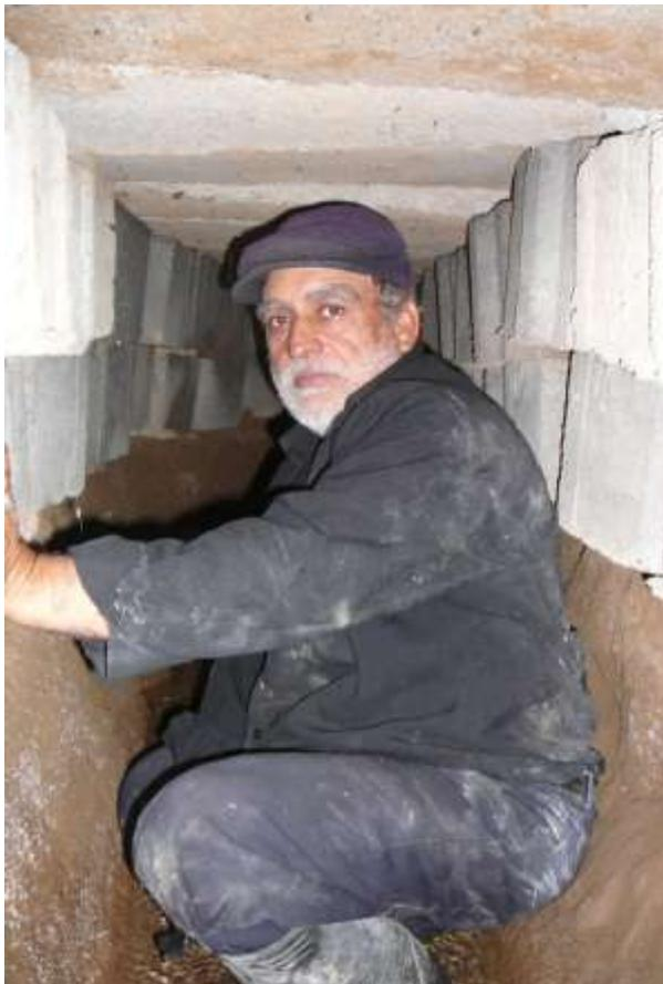
*Figure 3 a: The initial section of the qanat I went down. The lower part is old, the upper reinforced by concrete blocks. Image ©Caroline Mawer 2009*
